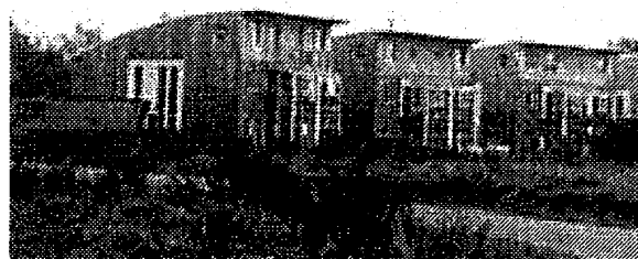
Fig. 3 Apartment houses installing Bio-gas system in Germany
